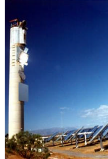
Solar Tower / Central Receiver
